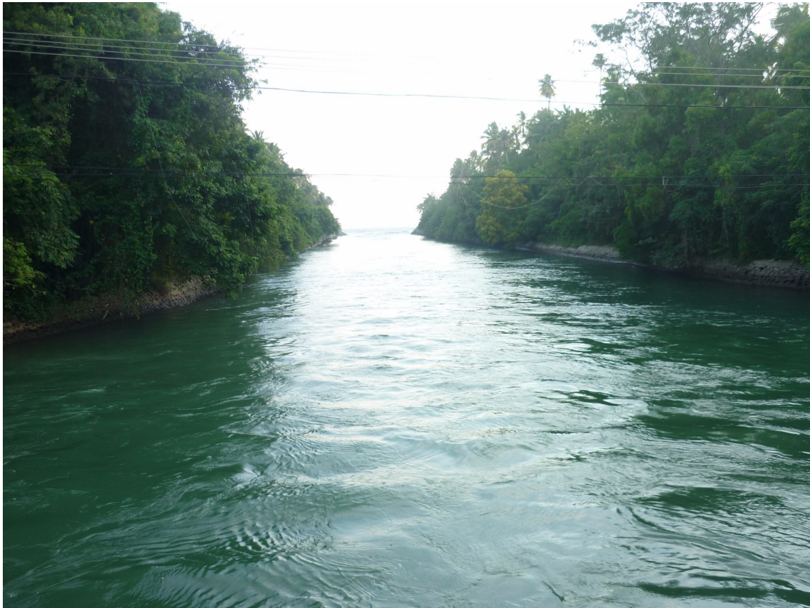
Figure 4: Spillway as seen from Paravur Lake
